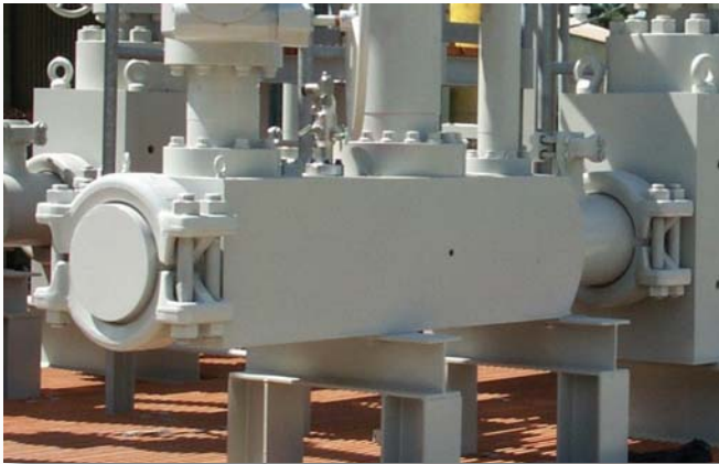
9" API 10000 psi "Building Block" Header
