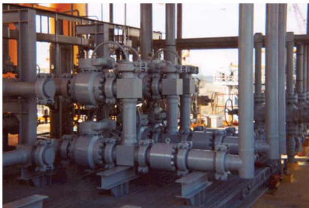
4.1/16" API 15000 psi "Building Block" Manifold
